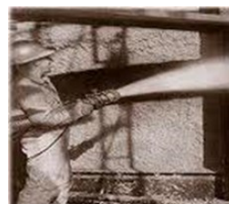
Spraying asbestos mix insulation on a structural steel work.
