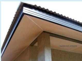
Asbestos cement sheet eaves lining.
