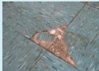
Asbestos floor tiles and adhesive.
