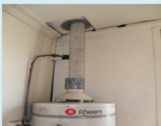
Asbestos cement flue left in place for new hot water system.
