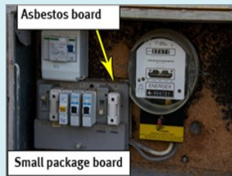
A small package board mounted over an asbestos insulation board or mill-board, (white material partially visible behind the package board is the asbestos board).
