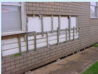
Simulated brick asbestos cement sheet cladding—moulded slices of brick attached to asbestos cement sheeting.
