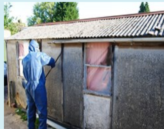
Old Garage & work shed with asbestos cement roof sheeting & asbestos sheet walls.
