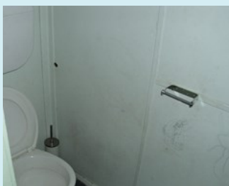
Asbestos cement sheet walls in a toilet.
